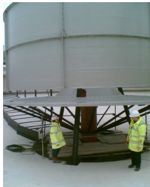
Figure 2: New Ø35m tank with MMI Designed McKinney baffle & deflection ring
