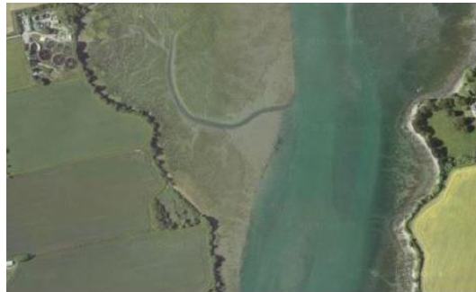
Figure 1: The source of sea water at the works is a result of seawater ingress into the sewer system
