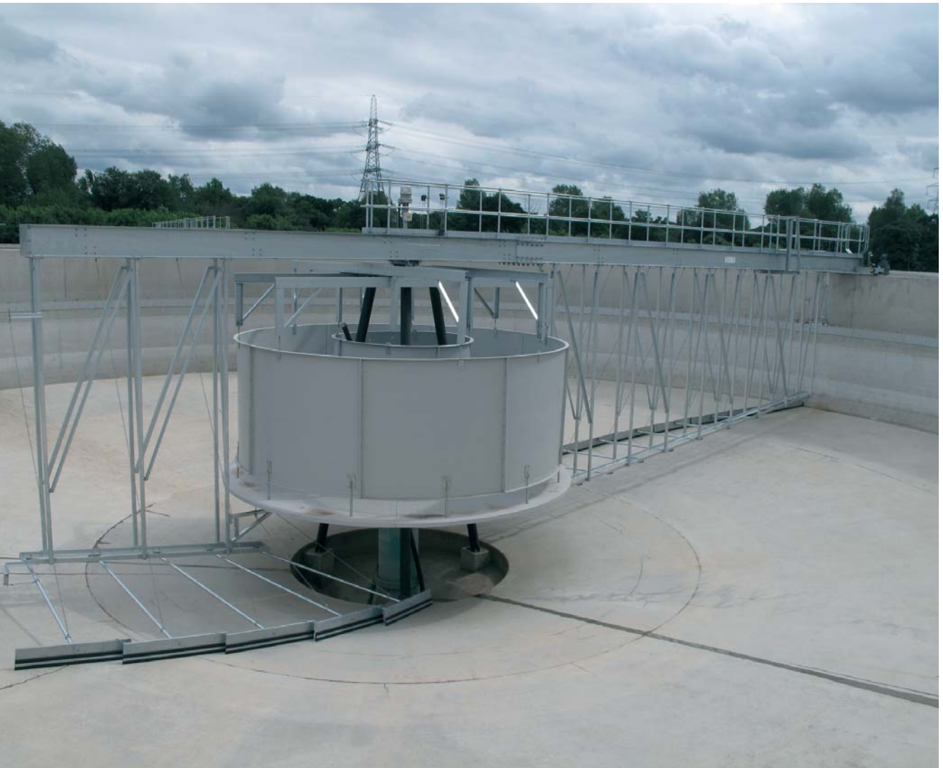
First ¾ Bridge for large diameter FST
