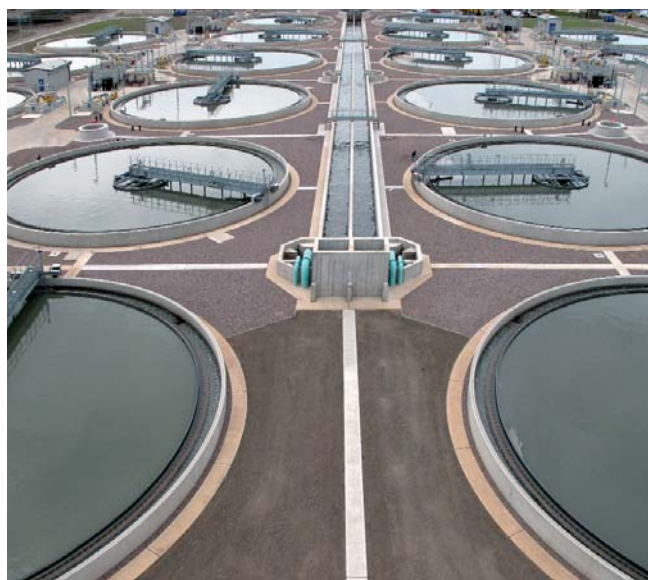
Primary Tank Island and Culverts
