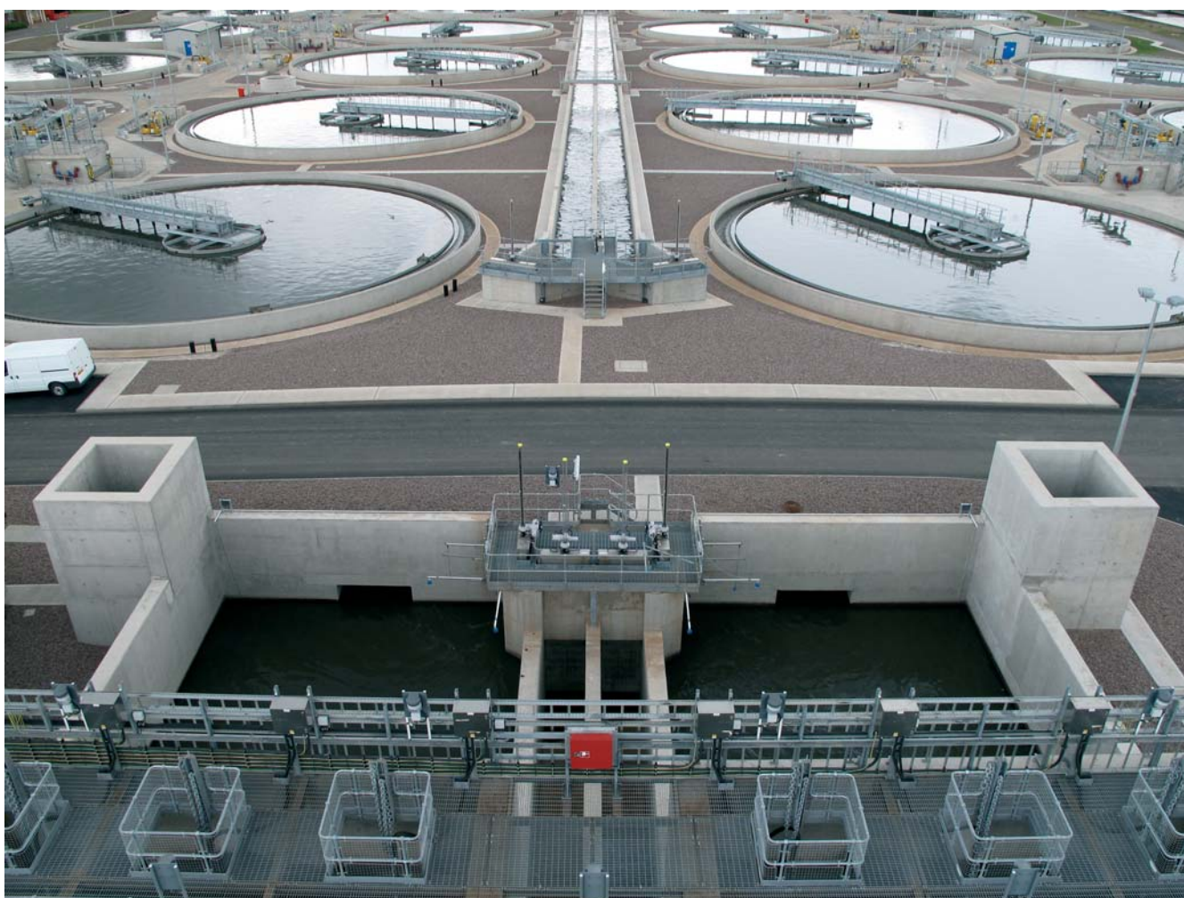
Minworth STW: Settled Sewage Pump Station (front) and Primary Tank Island (rear)
