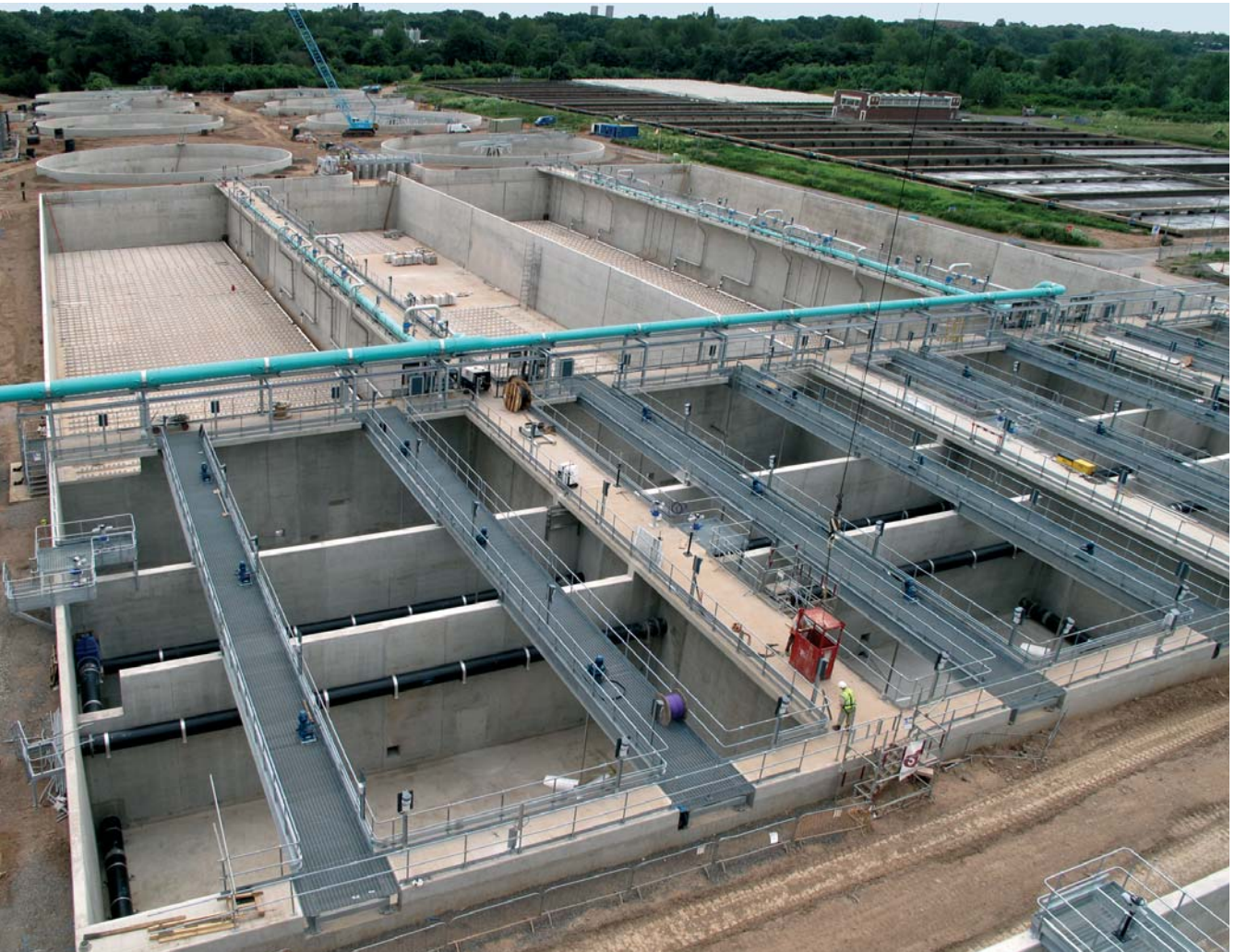
ASP 7 Construction and M&E installation well advanced
