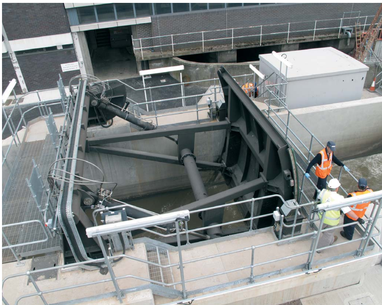
Innovative Radial Gate Flow Control Device
