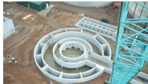
Figure 4: Chamber during construction (photograph courtesy of ukwaterprojectsonline.com)
