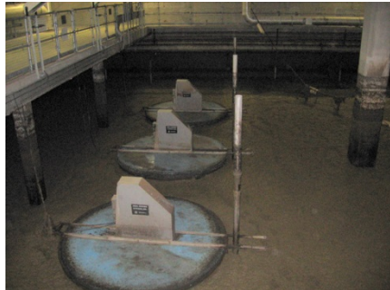
Figure 1: Surface Floating Decanters Weymouth SBR
