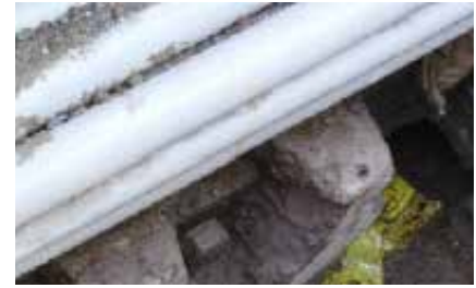
Excavations were undertaken to confirm condition of components
